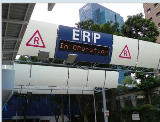
Picture 8: Automatic tolling gantry of Singapore's Electronic Road Pricing system in 2008
